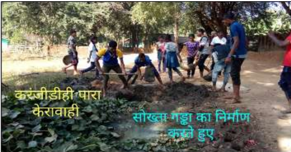
Fig.: NSS volunteers constructing Soak-Pit at Karanjdihipara of Kerawahi village.
